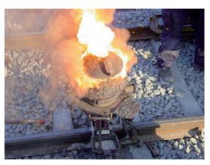
Figure 4.5 | The thermite reaction. Pictured here is a device for making white-hot iron by the reaction of aluminum with iron oxide and letting the molten iron run down into a mold between ends of two steel railroad rails. This welds the rails together. (Wikimedia Commons)
